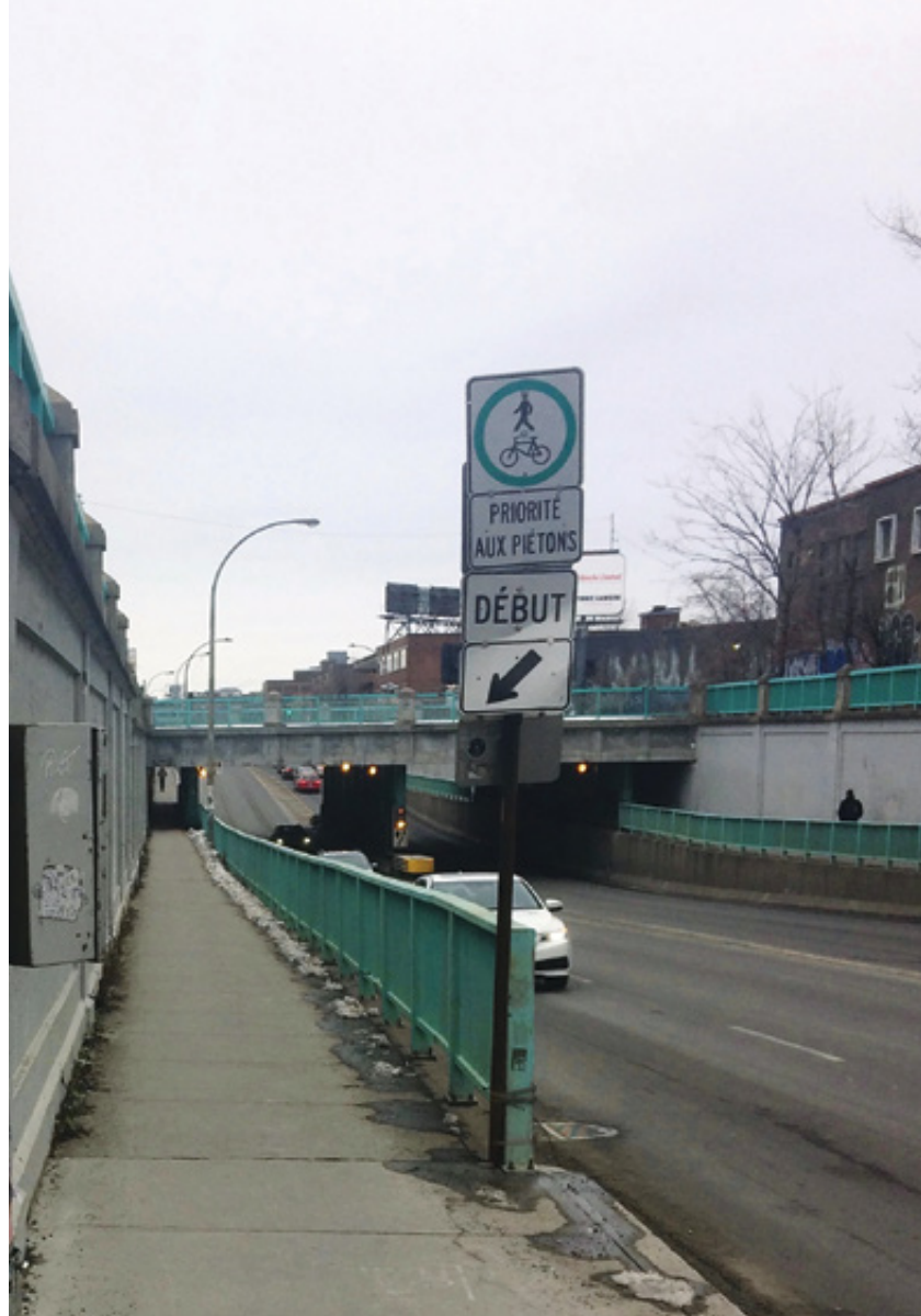
Cyclists and pedestrians must share the sidewalk on the Parc Ave. underpass.
