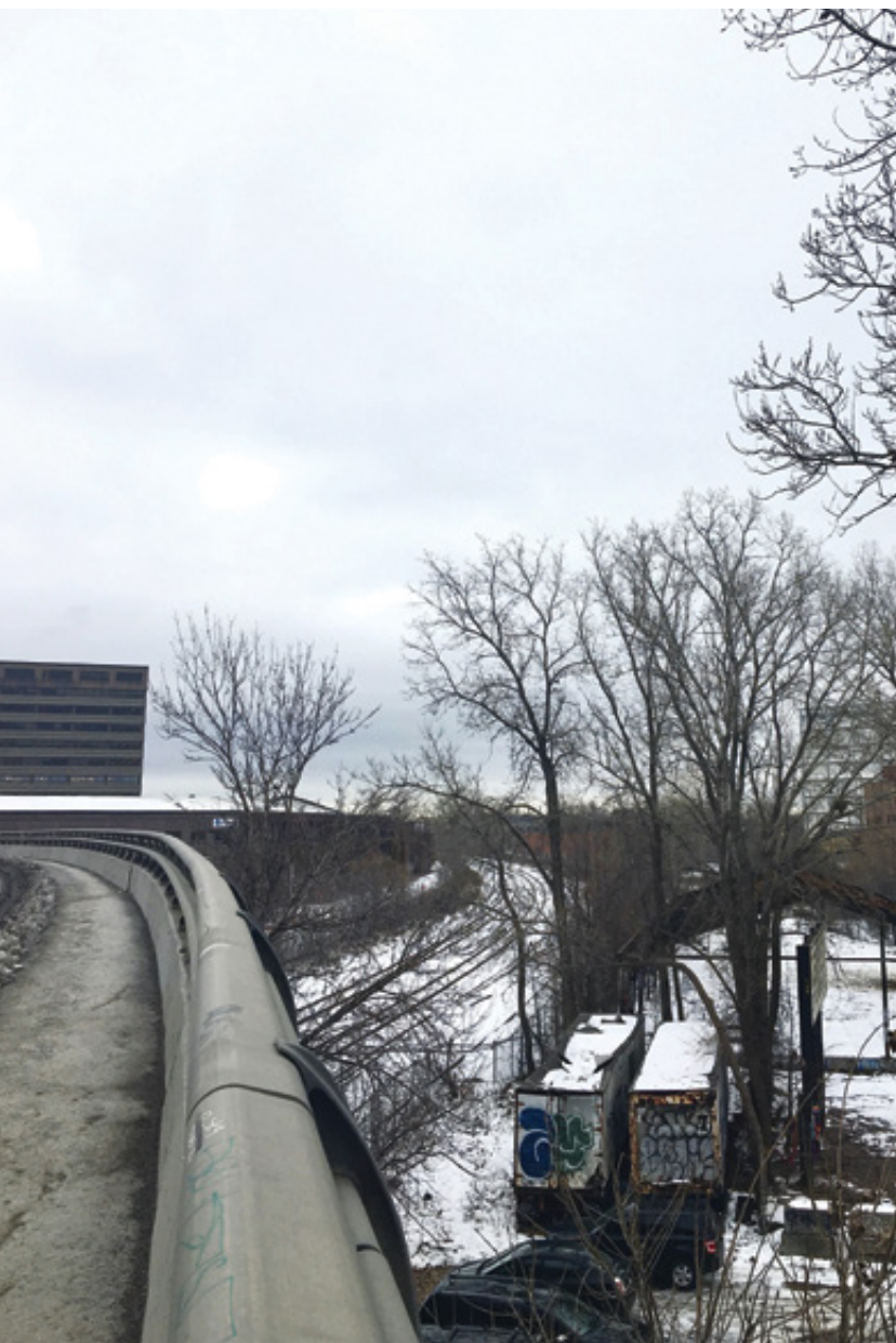
The skeleton of a torn down warehouse on the southeast edge of the tracks in Mile End.
